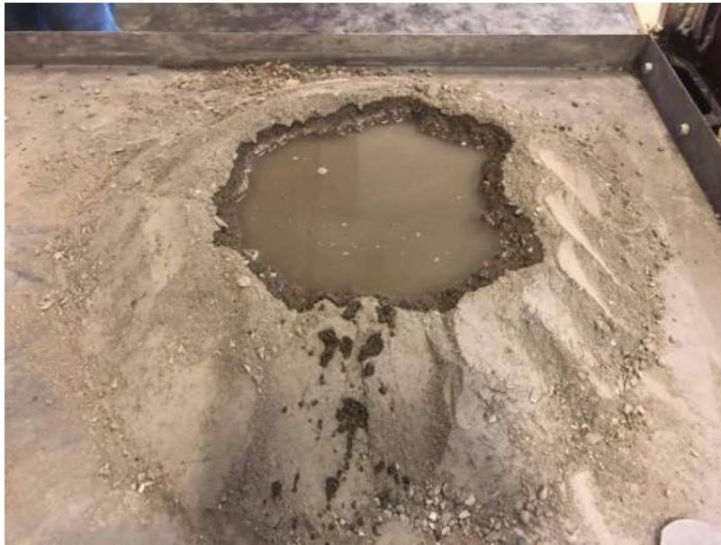
Figure 2: Mixing a batch of concrete.
